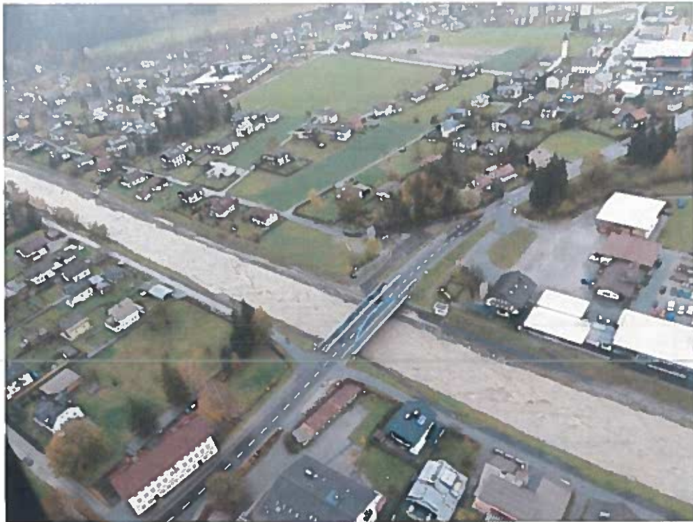
Photo 11: Gail in Kötschach-Mauthen (flood protection measures for HQ100)
