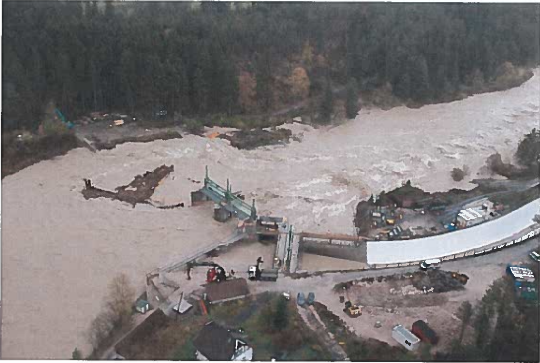
Photo 17: Gail at hydrological power plant Schütt (current construction site)
